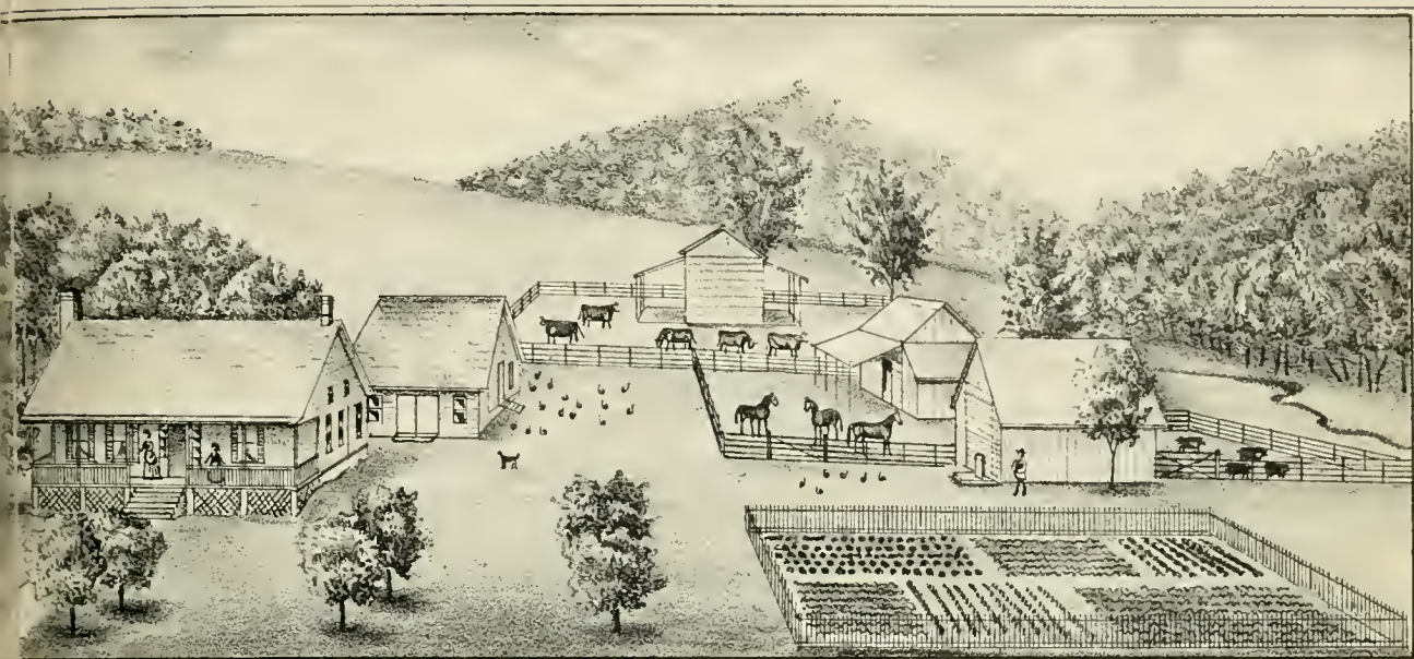
RESIDENCE OF PETER SNYDERS, SEC. 4. RICHWOODS PRECT. CALHOUN CO. ILL.
